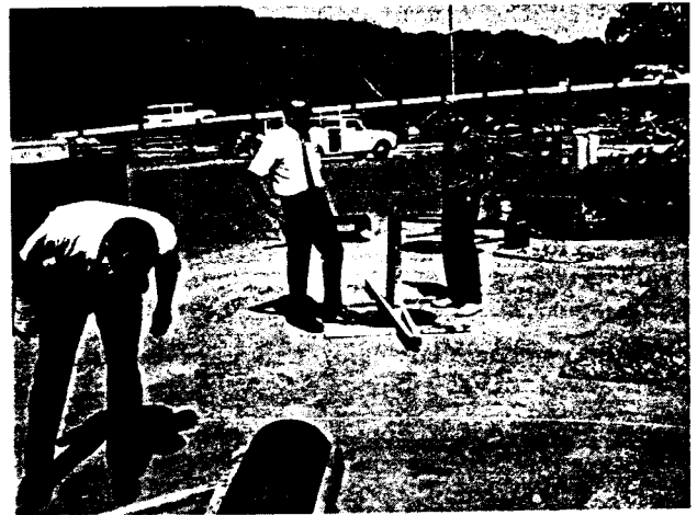
This was the SPEAR site in June of 1970, just after the initial foundation work had begun. From the left, Bill Davies-White, Bob Gould and John Rees check things out.
