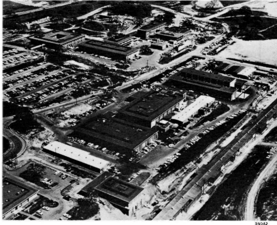
Figure 27-2 SLAC offices, laboratories, and shops.
