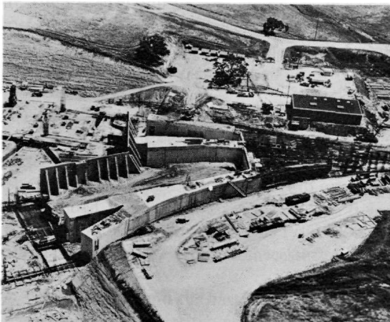
Figure 27-42 Beam switchyard nearing completion.
