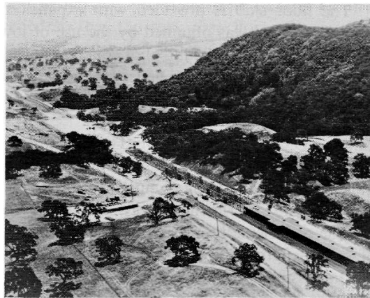
Figure 27-36 Klystron gallery under construction.
