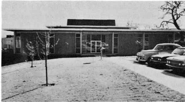
Figure 27-38 Central control building.
