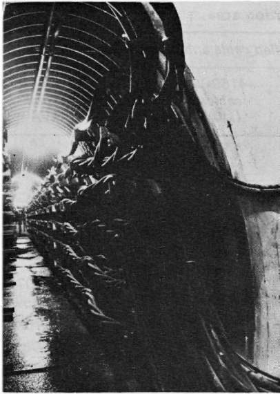
Figure 25-19 View from outgoing end of electrical utility housing serving utility vault.
